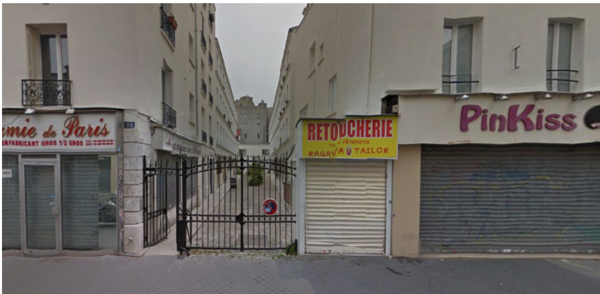
Rue Popincourt, Paris
